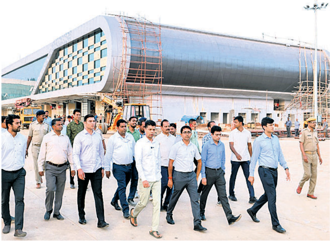
TAKING STOCK: 5T and Nabin Odisha Chairman VK Pandian reviews the ongoing work at Baramunda Inter-State Bus Terminal (ISBT) in Bhubaneswar, Friday. BDA Vice-Chairman Balwant Singh and City DCP Prateek Singh are seen
