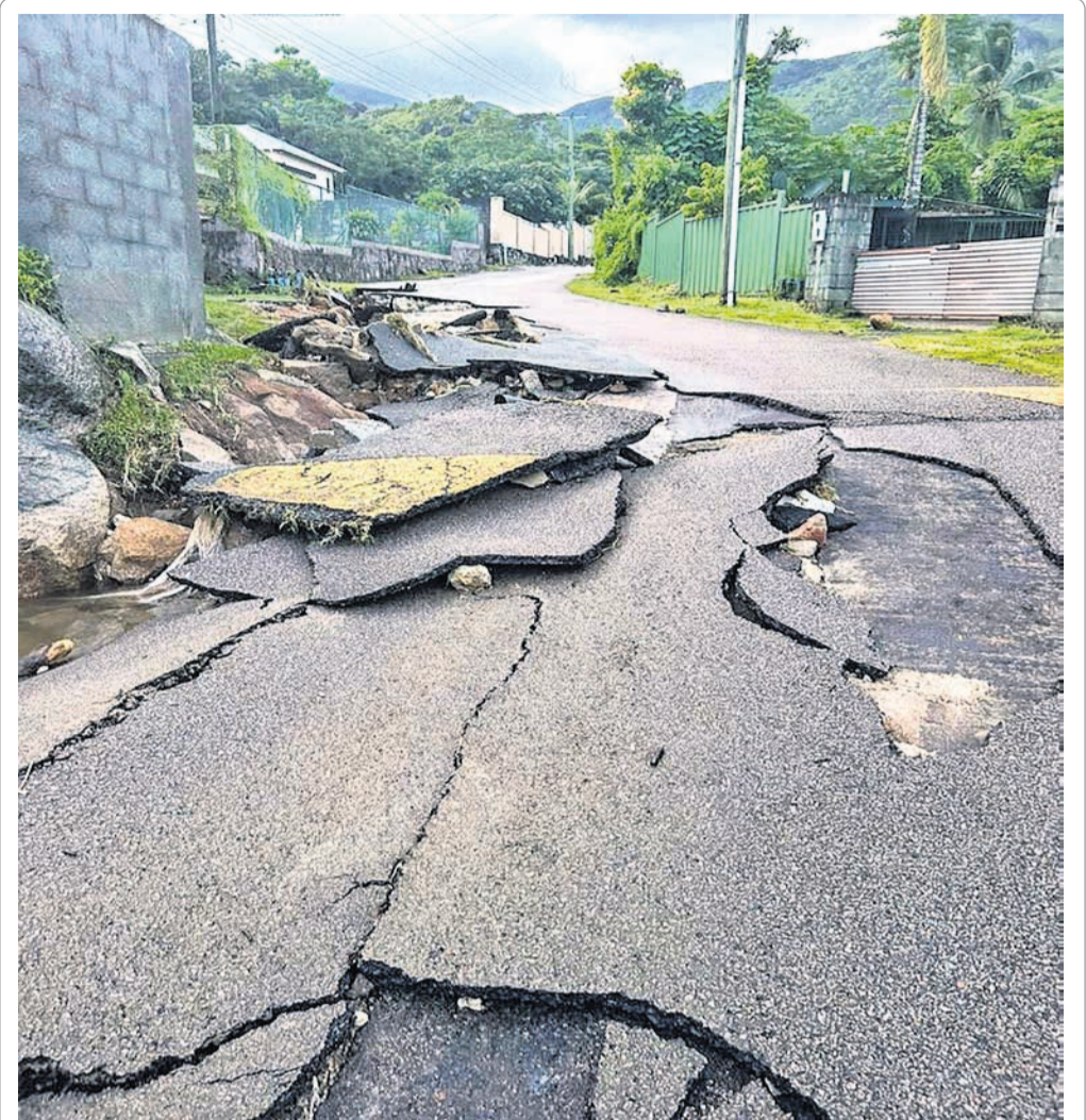
Cracks along a road in the aftermath of a massive explosion at an industrial area on the main island in Mahe, Seychelles, Thursday. Authorities in Seychelles declared a state of emergency Thursday after a blast at an explosives store caused massive damage in an industrial area also facing flooding amid heavy rainfall, according to the presidency
