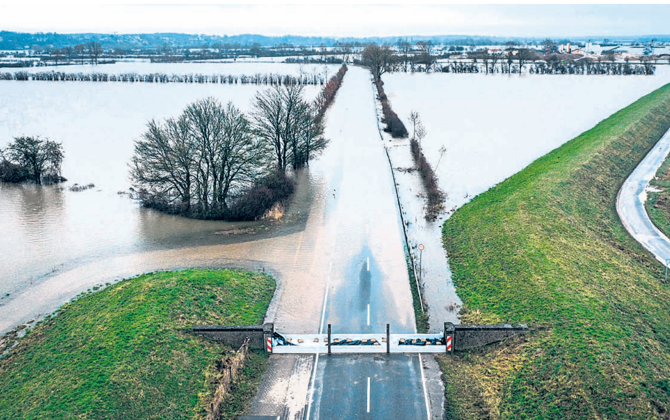
A flooded road is seen in Thedinghausen, Germany
