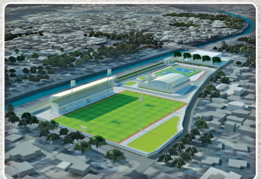
Football Training Centre Cuttack
