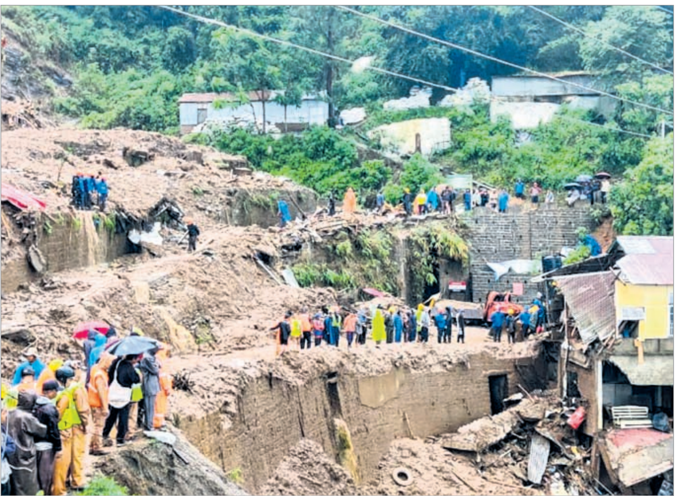
STORM AFTERMATH: Rescue work underway after a stone quarry collapsed amid heavy rain in Mizoram's Aizawl district, Tuesday. At least 25 people, including 14 in the collapsed stone quarry, were killed in the state due to landslides and incessant rain in the aftermath of cyclone 'Remal' (Report P3)
