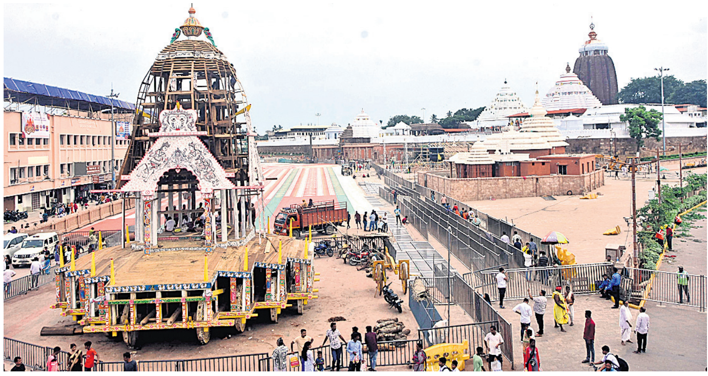
SETTING STAGE: Chariot construction reaches last leg on Grand Road in Puri, Wednesday
