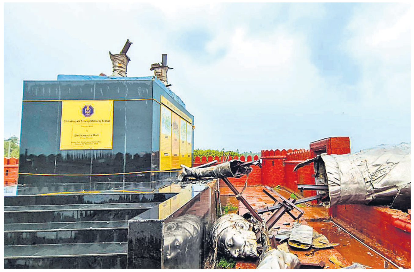
A statue of Chhatrapati Shivaji Maharaj, erected by the Navy and inaugurated by Prime Minister Narendra Modi last year, collapses at Rajkot Fort, in Malvan, PTI PHOTO
